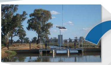
Automatic gates are connected to a SCADA package for remote monitoring and control, generating real channel performance data.
